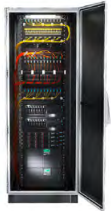
Rittal TS IT Server Cabinet Image courtesy of Facebook
